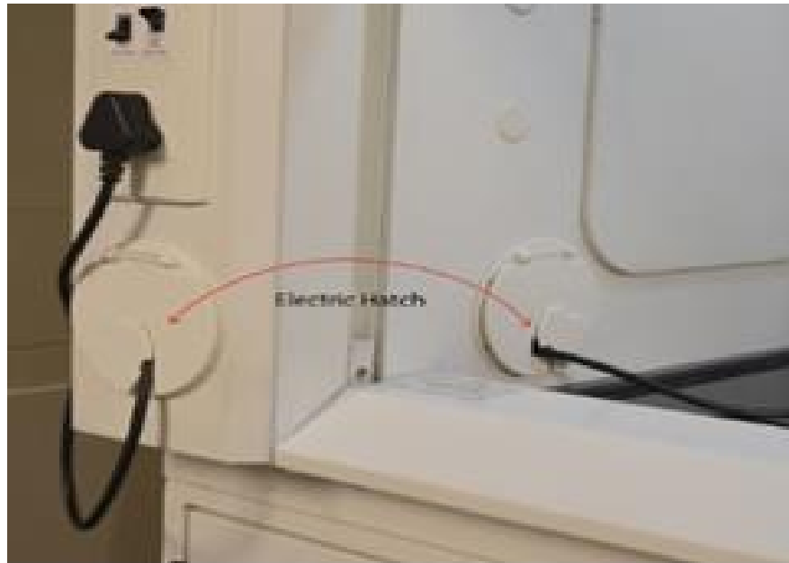
FIG: 16 TYPICAL ELECTRICAL HATCH DETAILS
