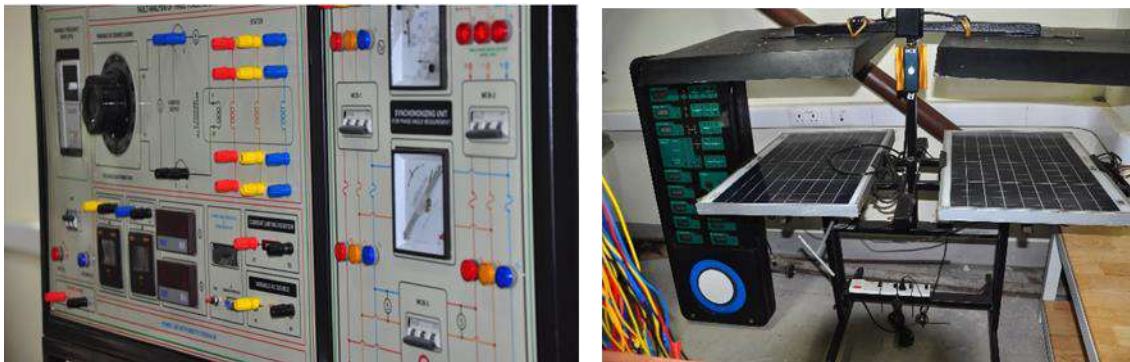
Power Systems Lab, Left: Alternator Fault Simulator wWith Grid Synchronization Facility, Right: Solar Photo Voltaic Array Simulator
