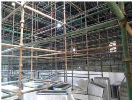
Auditorium work in progress
